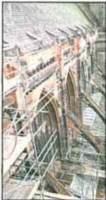
The Lady Chapel is undergoing major restoration work. (AK200210-0210A)
