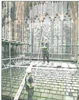
Workmen assemble scaffolding. (CS170409-3910LM)
