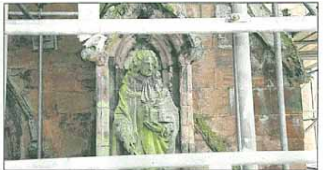
Sir Christopher Wren's statue, surrounded by scaffolding. (CS170409-3012LM)
